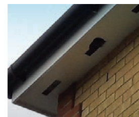
Typical parakeet access points around buildings in South London – one vent hole has been enlarged.
