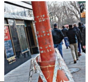
Some streets have district heating pipes in or near the sewers. There the rats are abundant. You can see the orange chimneys everywhere.
