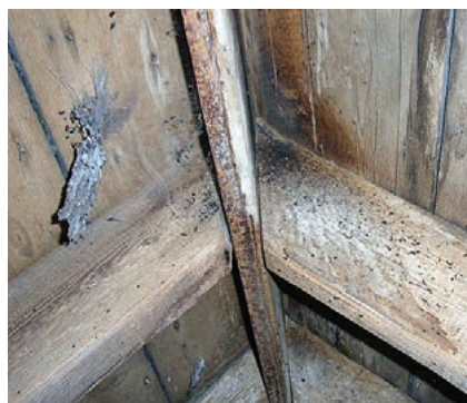
Staining and droppings indicate the presence of bats (image: BCT/John Haddow)
