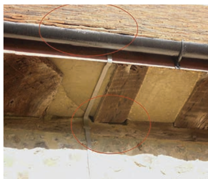
Potential roosting and access points in historic building with bat roost (image: BCT)
