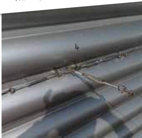
Figure 2: perimeter wire ropes each anchored using a pair of angle brackets and a central cross wire where the tension pulls the screws sideways rather than directly out of the cladding.
