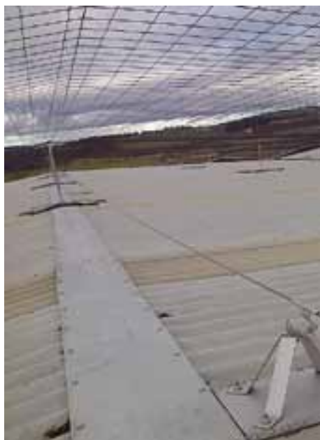
Figure 1: network roof mounts with 2m net support pole.
