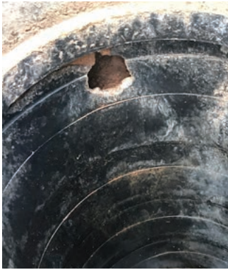
Typical rat damage to the wall of an inspection hatch
