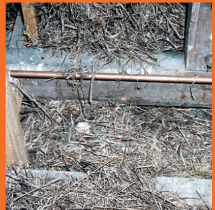
Attic nest debris from the case study (pg21)
