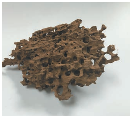
Deathwatch damage to a section of timber
