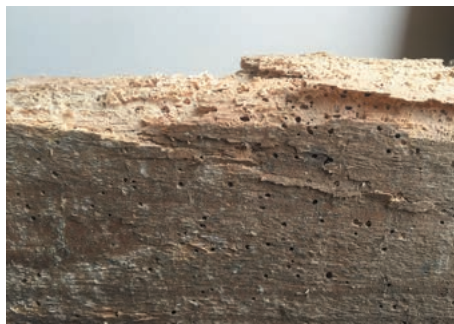
Common furniture beetle damage to timber
